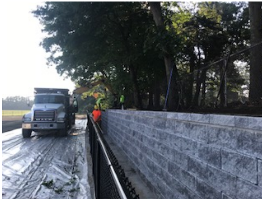
Multipurpose Field Retaining Wall And Fence
